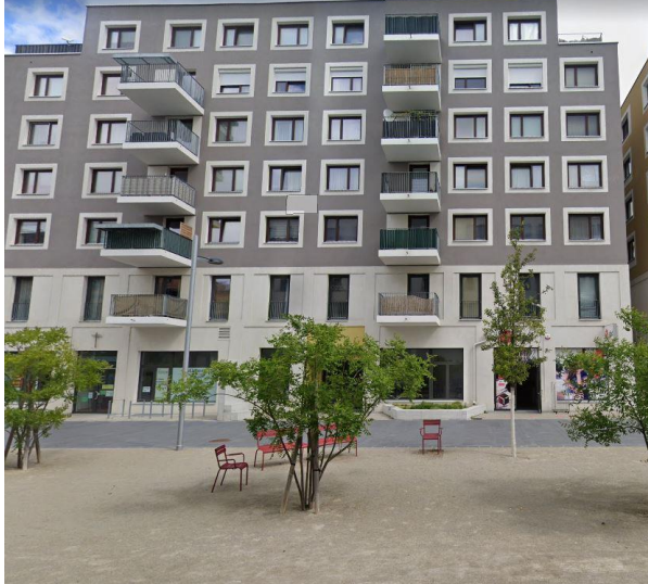
The balconies are too small and too high → shall be omitted.
