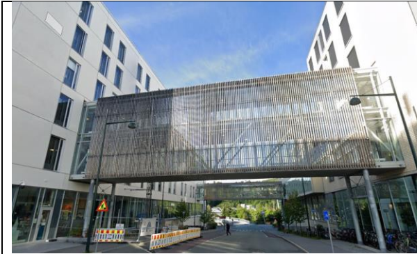
Bridges between buildings are placed in the field of view of the competitor → canopy.
