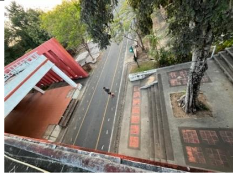
Multi-Level Buildings / Walkway.
